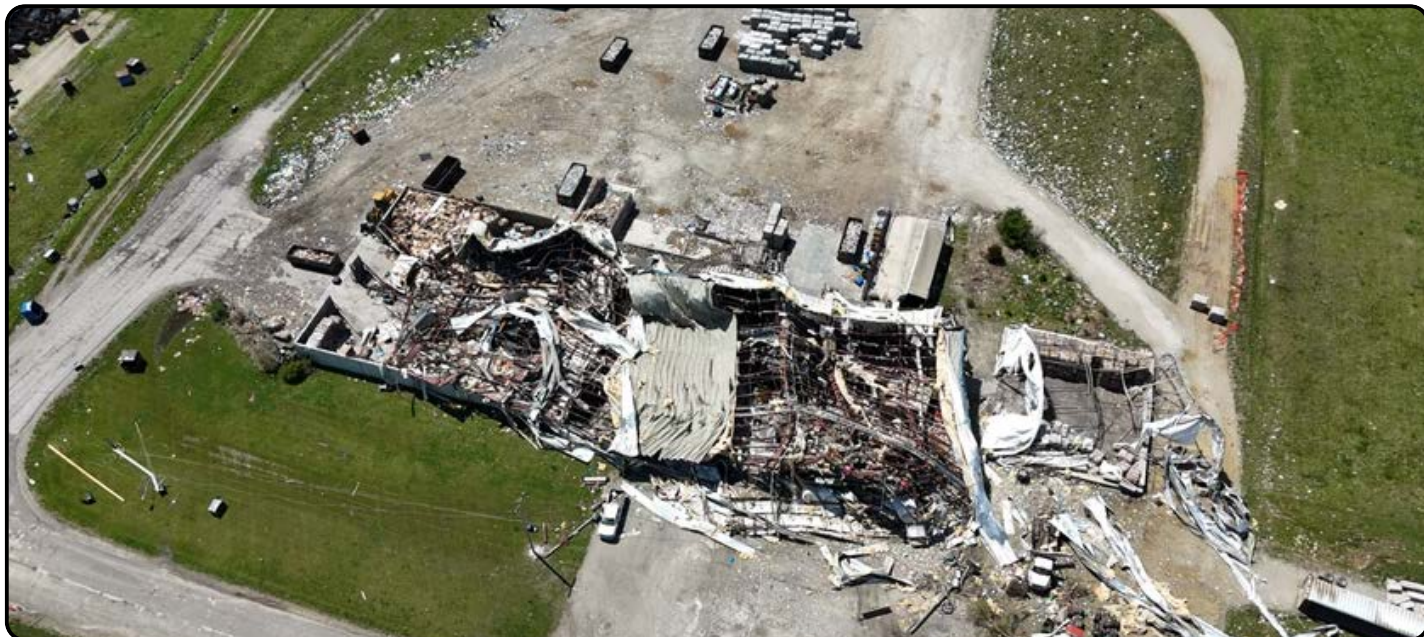
Photo: Aerial footage of the damage to the City of Columbia Materials Recovery Facility, located at 5700 Peabody Road (Photo attributed to KOMU 8).
